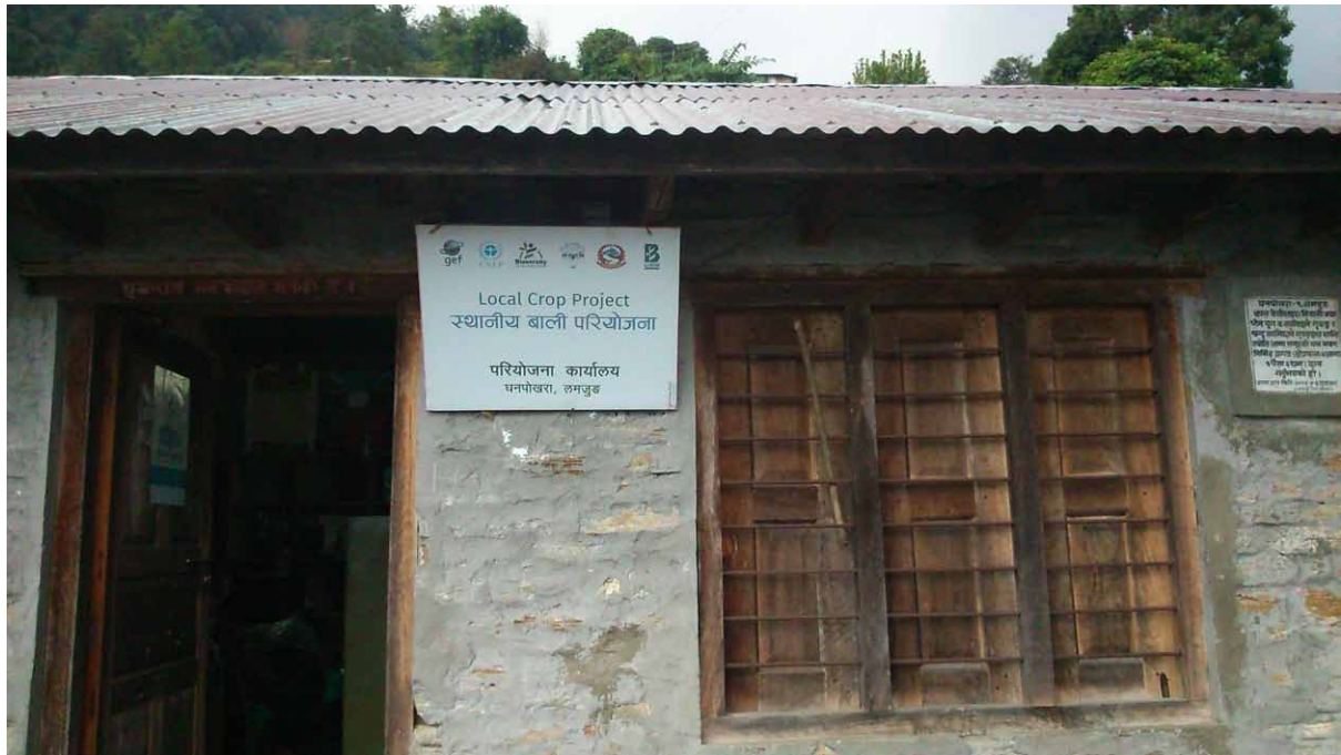
Figure 4: The newly built LCP office in ward #1
